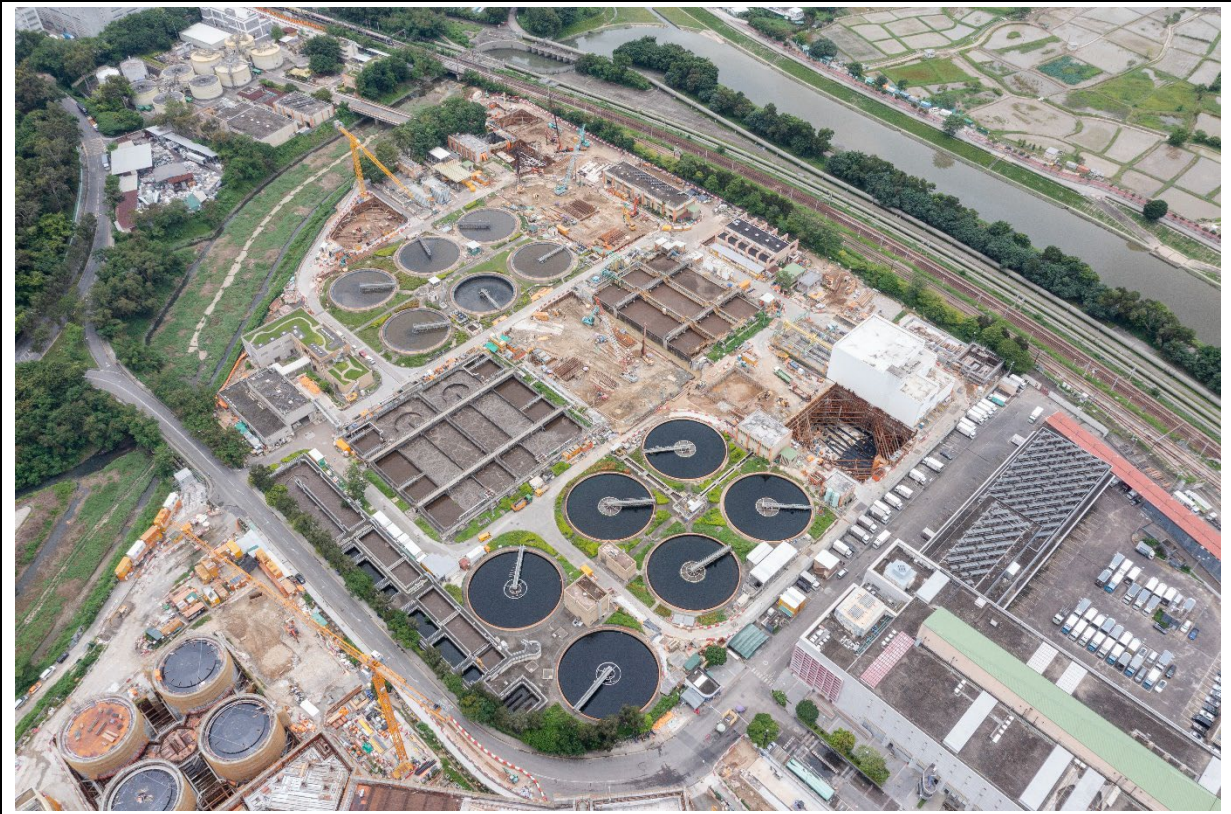
Description: Aerial Photo No. 1 in Portion A & Portion B on 20 June 2022
