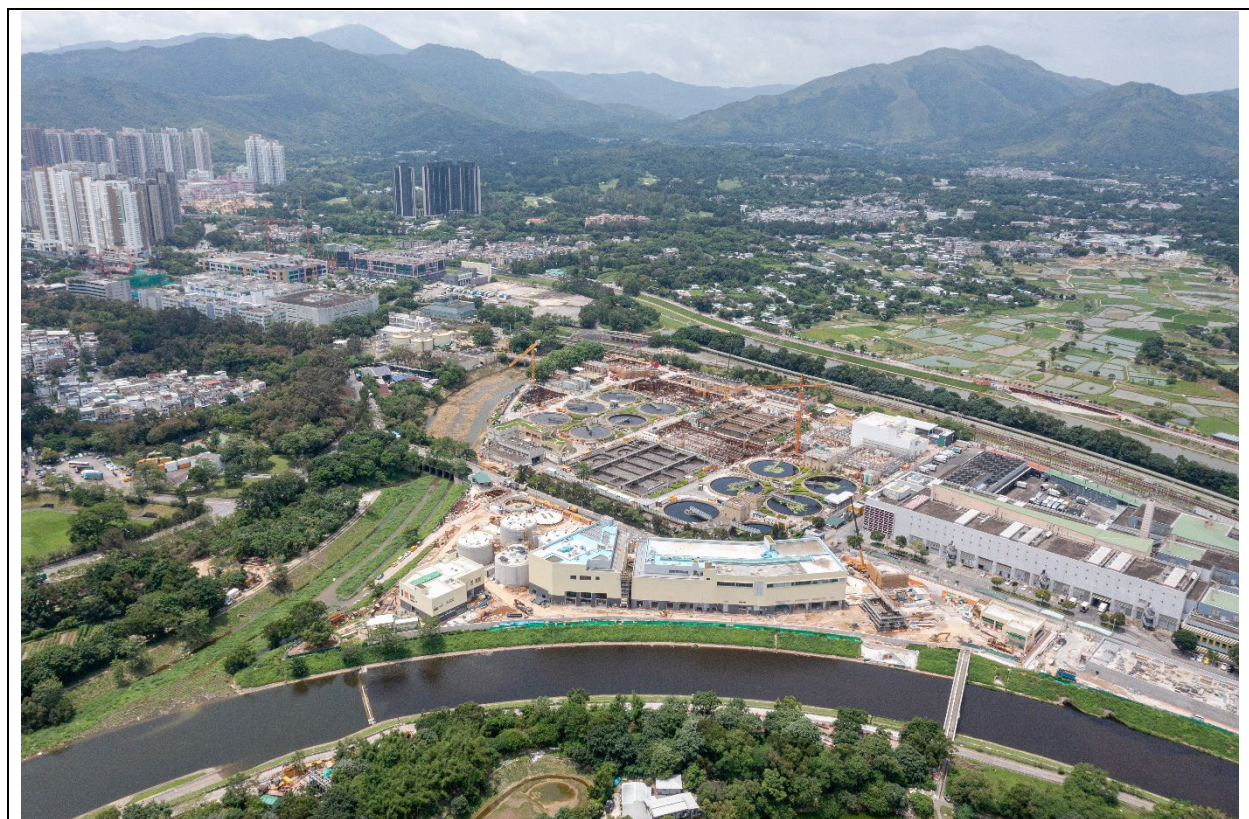
Description: Aerial Photo No. 2 in Portions C on 22 May 2023
